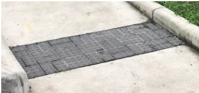
Clarity in crosswalk marking. ADA warnings
